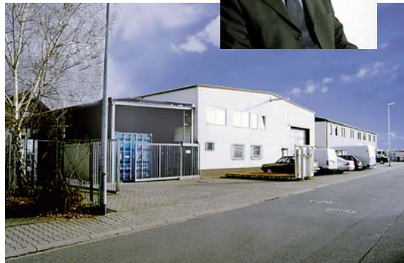
Main Office Herborn GmbH (Ginsheim-Gustavsburg, Germany)
